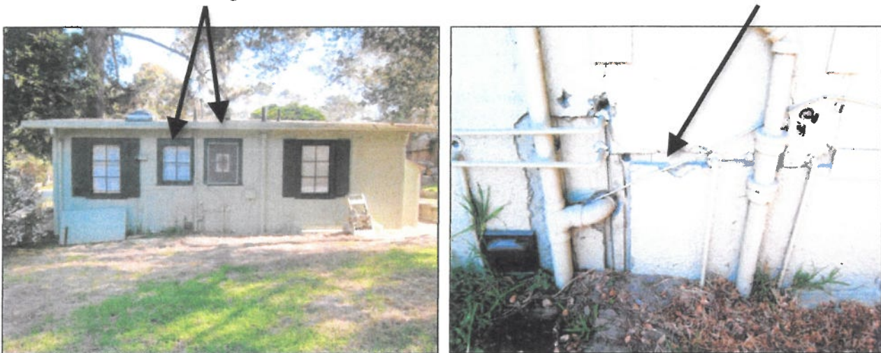
Figures 3 and 4. Left image shows the right side elevation with newer window inserts (arrows). Right image details the right side elevation and shows the Beaverboard siding, overcoated with a stucco finish and covering the original vertical board siding.
